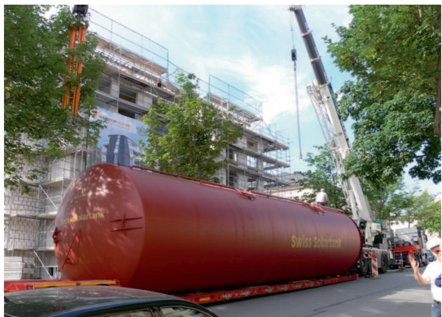
The core component of the building’s heating system is a 72 m<sup>3</sup> steel tank, incorporated into the base build in October 2020. With a diameter of 2.3 m and a height of 17.8 m, it extends to all floors of the house.
