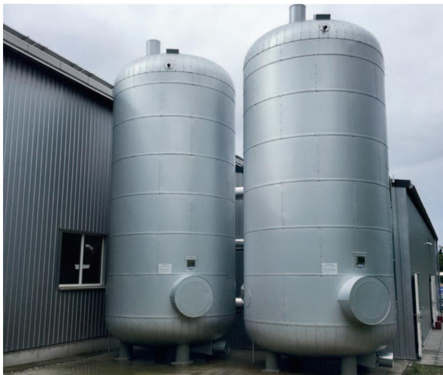
The two buffer storage tanks in Breklum have a volume of 44 cubic meters each.
