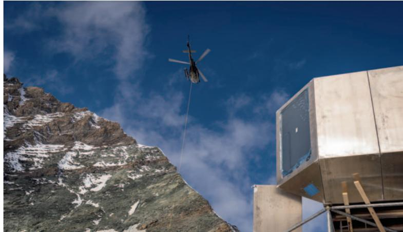
Helicopters flew all the prefabricated hut components to the construction site - including the module with the integrated solar air collector, which can be seen at the front in the picture above.
