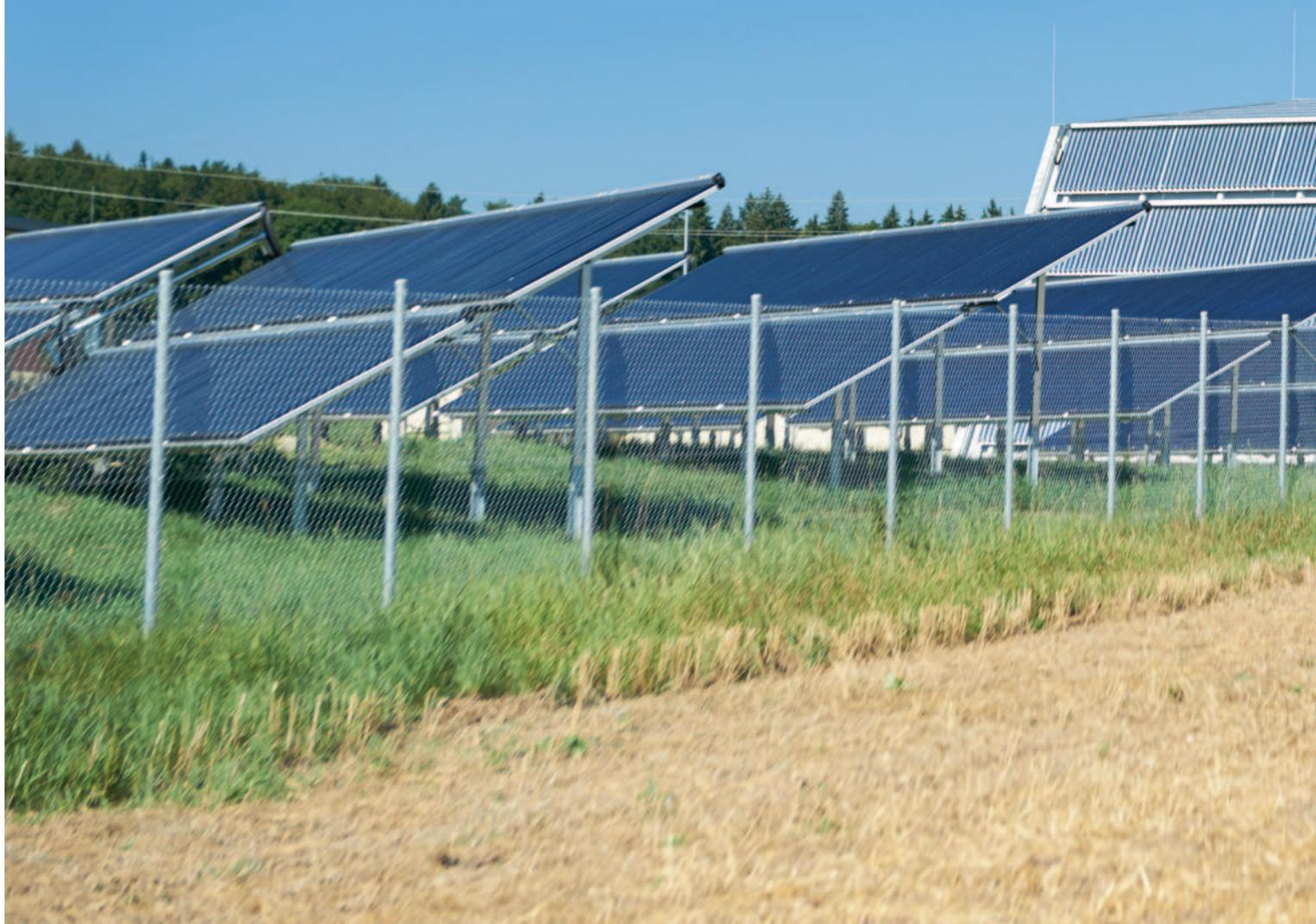
The installation of central solar heat supply systems can achieve the heat turnaround more quickly than installations on each individual house. For this reason, the Ritter company began planning and installing solar systems for district heating networks at an early stage.
