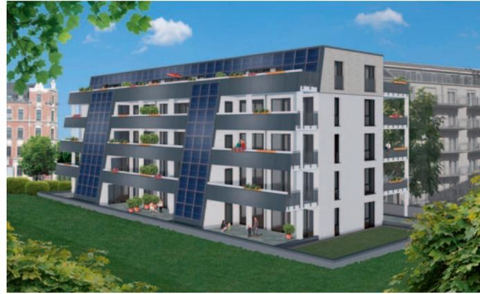
Garden view of solar domicile III (top): 340 square meters of solar collectors installed in February 2021 (bottom) generate heat for 24 condominiums.
