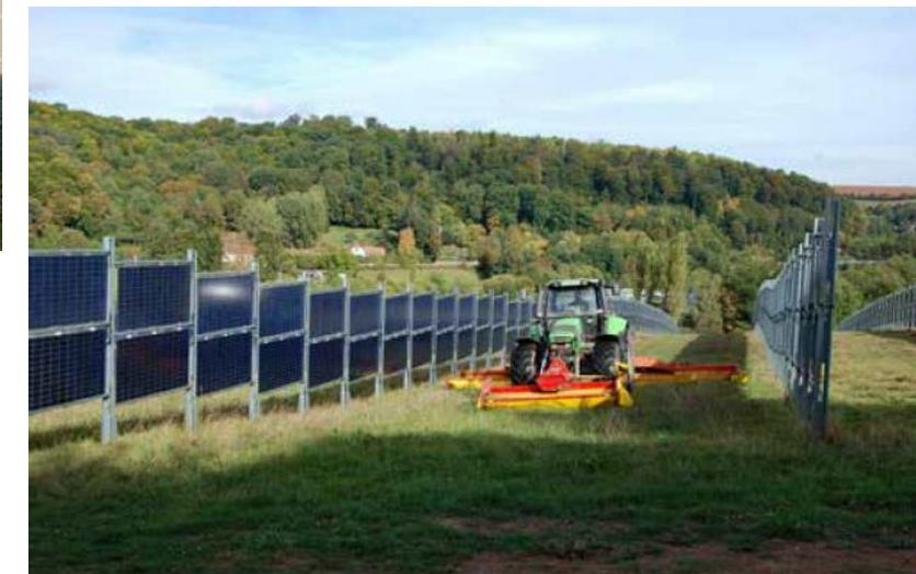
Impianti con moduli fotovoltaici bifacciali montati verticalmente su strutture fisse in the Eppelborn-Dirmingen solar park, Saarland, with 2 MWp capacity, constructed by Next2Sun GmbH. © Next2Sun GmbH
